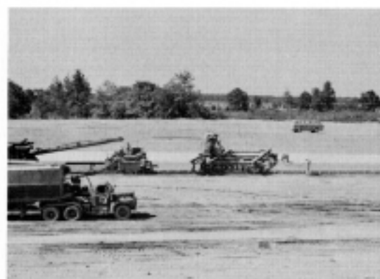
General View of Concrete Laying Operation - 2000 ft per day was normal paving.
