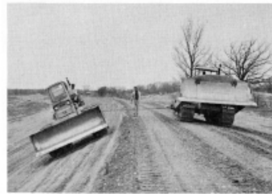
Compacting Sand Cushion
