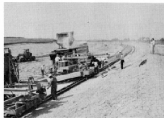
Spreading Concrete - Lane 4
