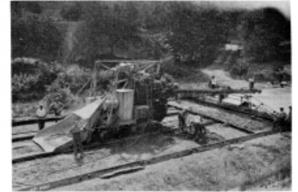
Laying concrete on straight section of Oval Test Track - 300 ft per day was considered very good.
